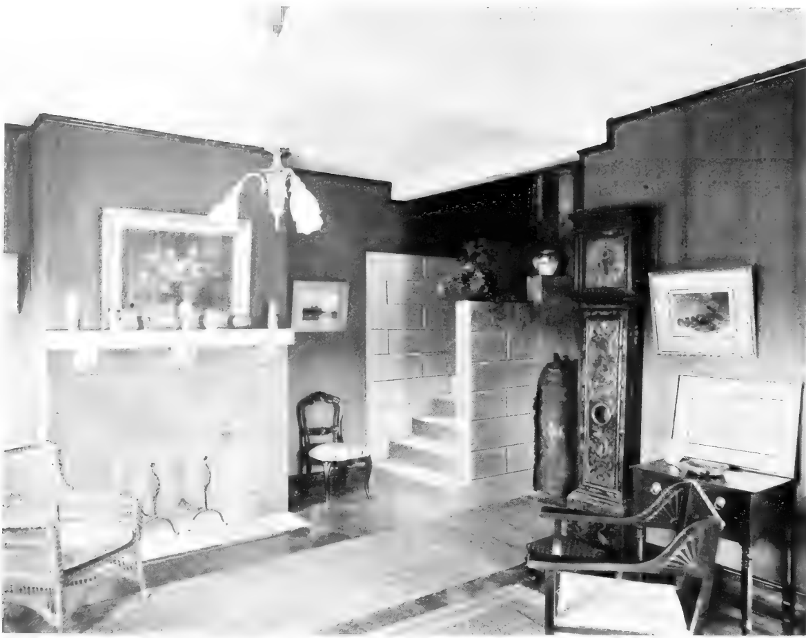
18 The Mantel and Shelf Supported on Corbeled Brackets is Built of Concrete. The Walls are Covered with Crimson Burlap. View Shows Reinforced Beams in Ceiling Which Carries the Floor Above
